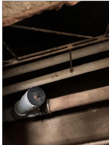
Asbestos-containing Aircell pipe insulation.
