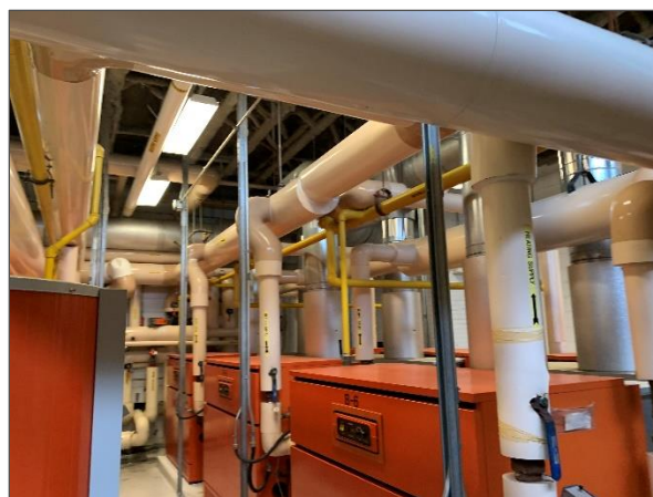
Non-asbestos insulated boilers.
