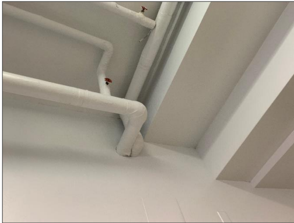
Asbestos-containing parging cement insulation present on pipe elbows.
